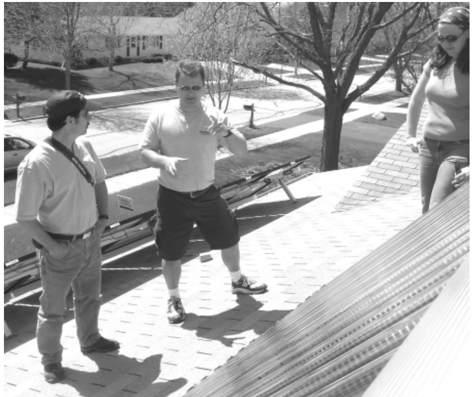
Jeff Riggert (center) stands on the roof of his net-zero-energy home and explains the workings of an evacuated tube solar water heater to Ross DePaolo (left) and another visitor during an open house in April.
