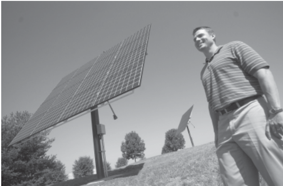
Two photovoltaic solar panels have been installed at Wisconsin Public Power Inc.'s Sun Prairie headquarters. WPPI Energy Services Representative Kurt Pulvermacher says the two panels installed at the company's Sun Prairie headquarters will follow the sun's movements throughout the day to increase system's efficiency by as much as 30 percent.
