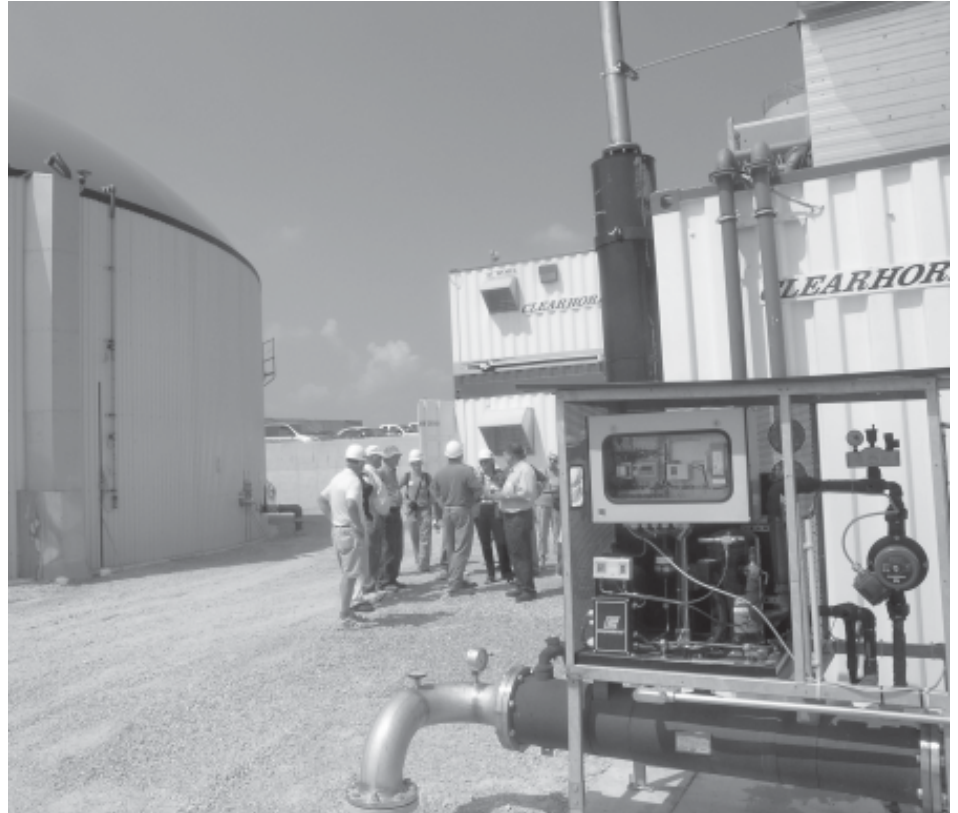
Crave Brothers Dairy Farm hosted open house to let visitors tour the new biodigester installation. Methane gas from the digester tank at the left travels underground and into a dryer in the foreground before powering a diesel engine and generator in the building behind the dryer.
