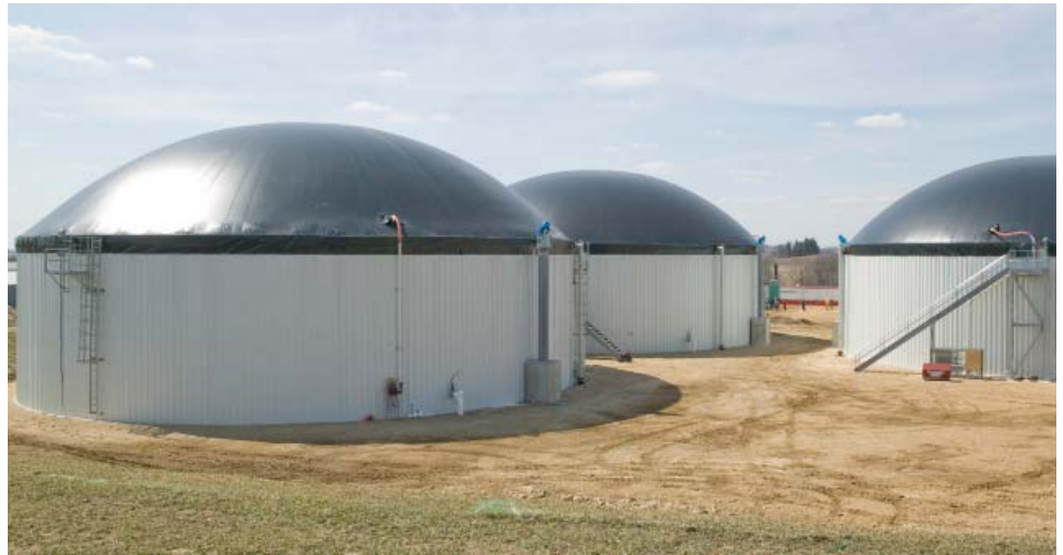
Three tanks store up to three million gallons of manure from three farms for digestion and electric generation at Dane County's community digester. Photo by L&S Technical Associates
