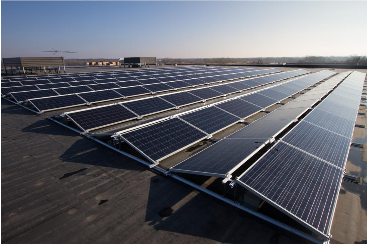
*SunPeak's DeltaWing™ mounting system was used, which features an east/west module orientation. This low profile design not only looks great, but reduces roof loading and provides more consistent power output. Energy density was increased 30% relative to south facing alternatives.*
