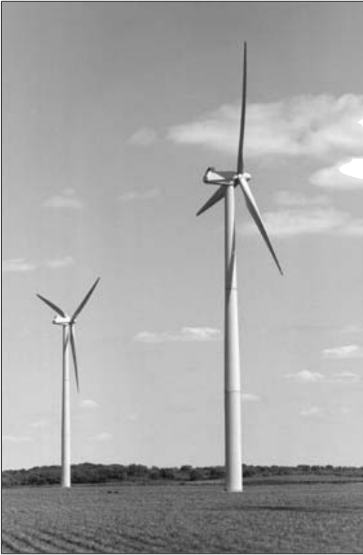
Typical Wind Generation Installation
