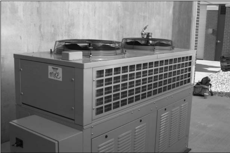
STM Stirling Engine/Generator (Beta version), 25 kW External View
