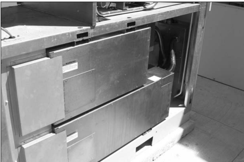
Capstone MicroTurbine Inverter Assembly
