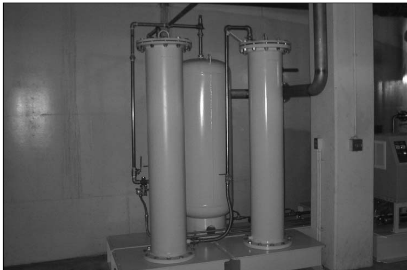
Typical biogas siloxane removal system
