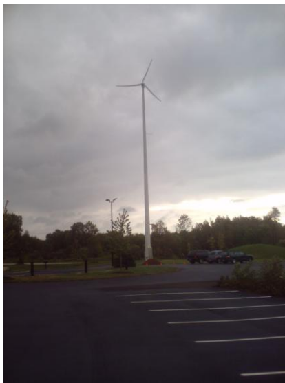
Small Wind Turbine
