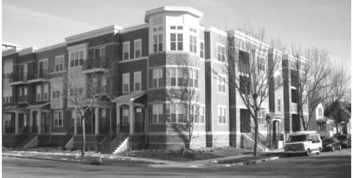
COURTESY OF ENERGY CENTER OF WISCONSIN
