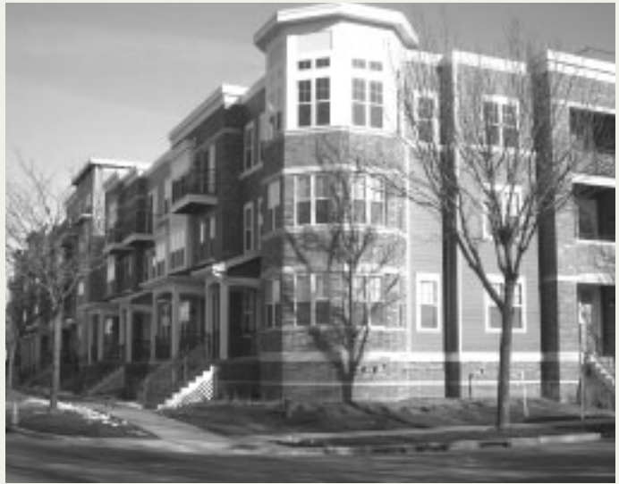
COURTESY OF ENERGY CENTER OF WISCONSIN
